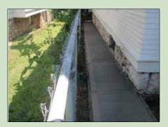
Many older homes in the zone have drainage problems due to cracked or damaged sidewalks that direct stormwater runoff towards foundations and basements. After receiving training, Community Crew members can repair and replace damaged sidewalks, sloping them away from foundations.
